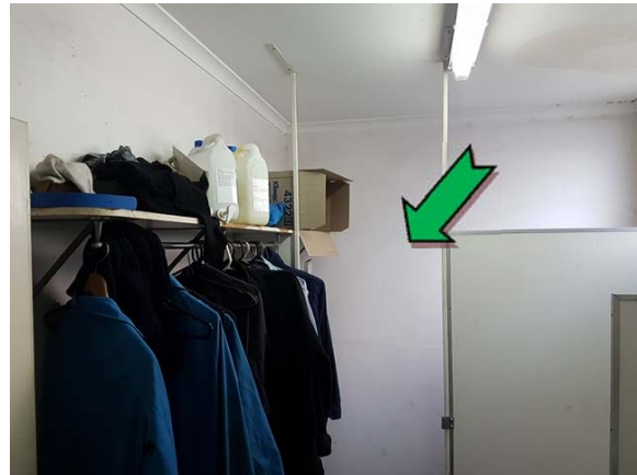
Photo 4. Interior, ground level, bathroom, walls – non asbestos-containing fibre cement sheeting.
