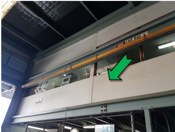
Photo 3. Interior, above kitchen, southern wall – assumed non asbestos-containing fibre cement sheeting.
