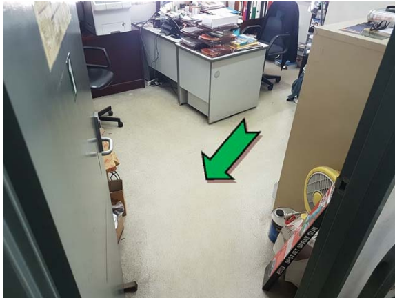
Photo 1. Interior, mezzanine level, western office, floor coverings – non asbestos-containing vinyl floor tiles.
