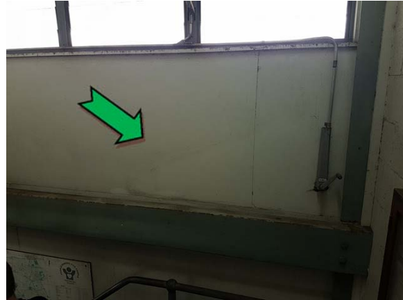
Photo 2. Interior, stairwell, walls – non asbestos-containing fibre cement sheeting.
